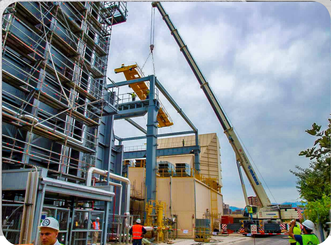
Erection of crane on steel structure
